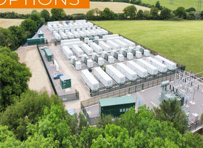
The largest unsubsidized grid-connected standalone battery storage plant in Europe: 100MW/100MWh Energy Storage plant at the 400kV UK national grid substation in Minety, UK.
